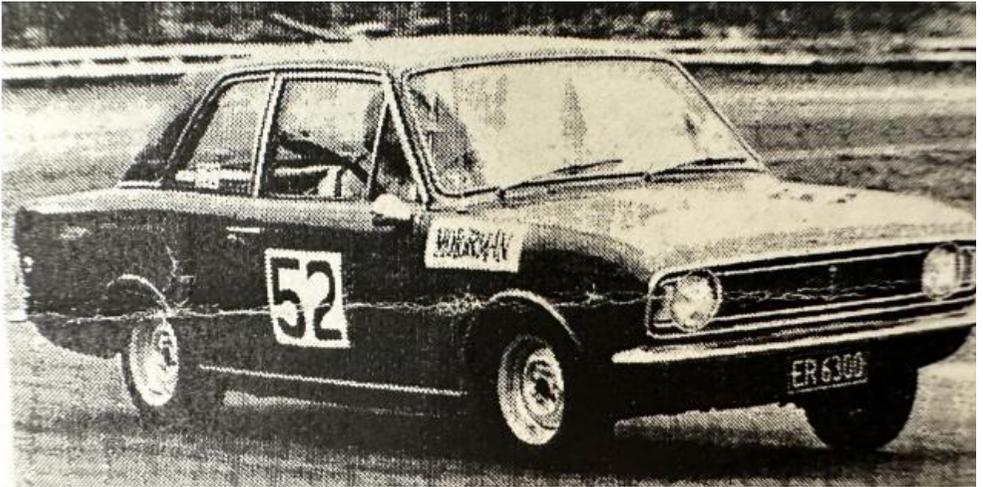
*Donn Anderson in the relatively plain Ford model at Bay Park raceway 1970. By this time there was no aluminium lightweight panels, a more conventional suspension in the rear, normal fuel tanks, and the new slightly larger Mark 2 body.*
